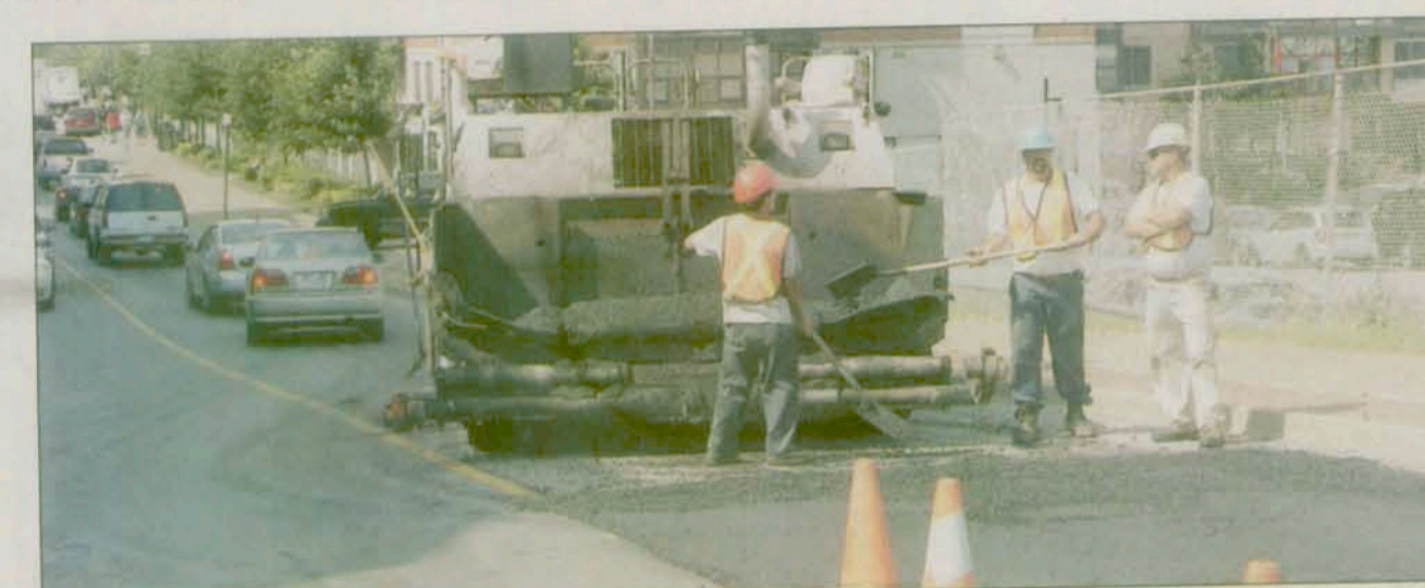
Workers apply new asphalt on a section of Lower Water Street in Halifax last summer.
